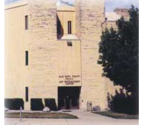
The Blue Earth County Jail
